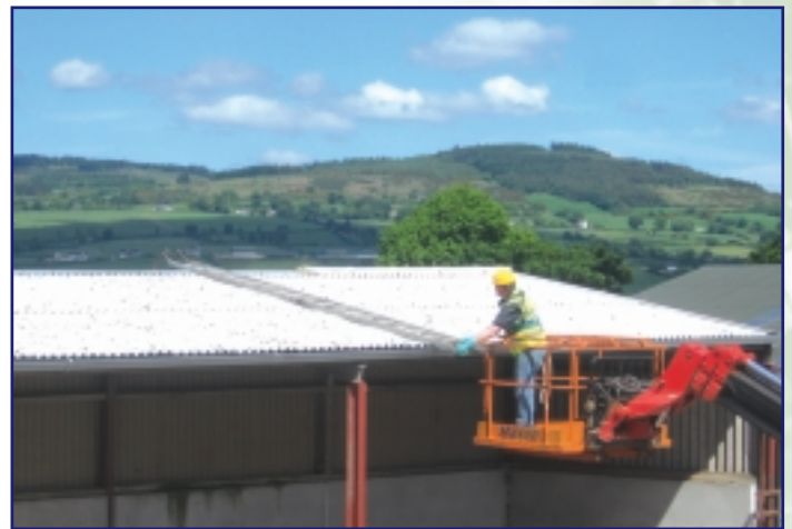
Elevated work platforms should be used safely
